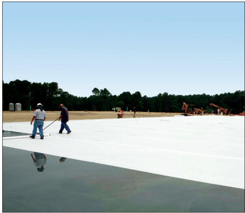
Wet curing covers are becoming popular. This curing method is the optimal way to cure a slab and increase abrasion resistance.
